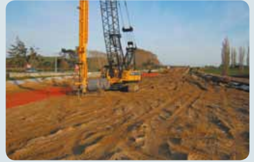
Over 15,000 wicks will be installed alongside SH2 to help drain the water content from the soft soil below.
