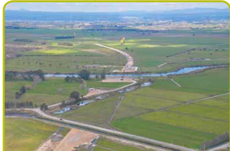
6 Location where TEL crosses Kaituna River heading east towards Paengaroa
